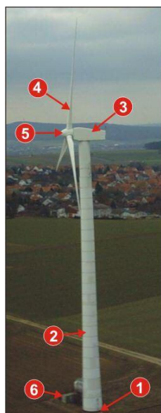
Figure 2 – Schematic view of the components of a wind turbine. (Source: WWEA, 2006 9 ).
