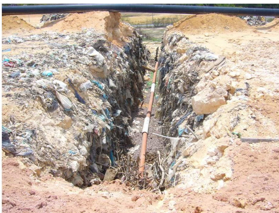
Figure 3 - Example of horizontal collection system (trench)
