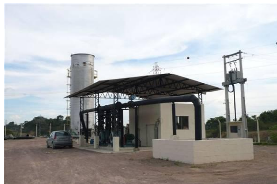
Figure 7 - Condensate knockout
