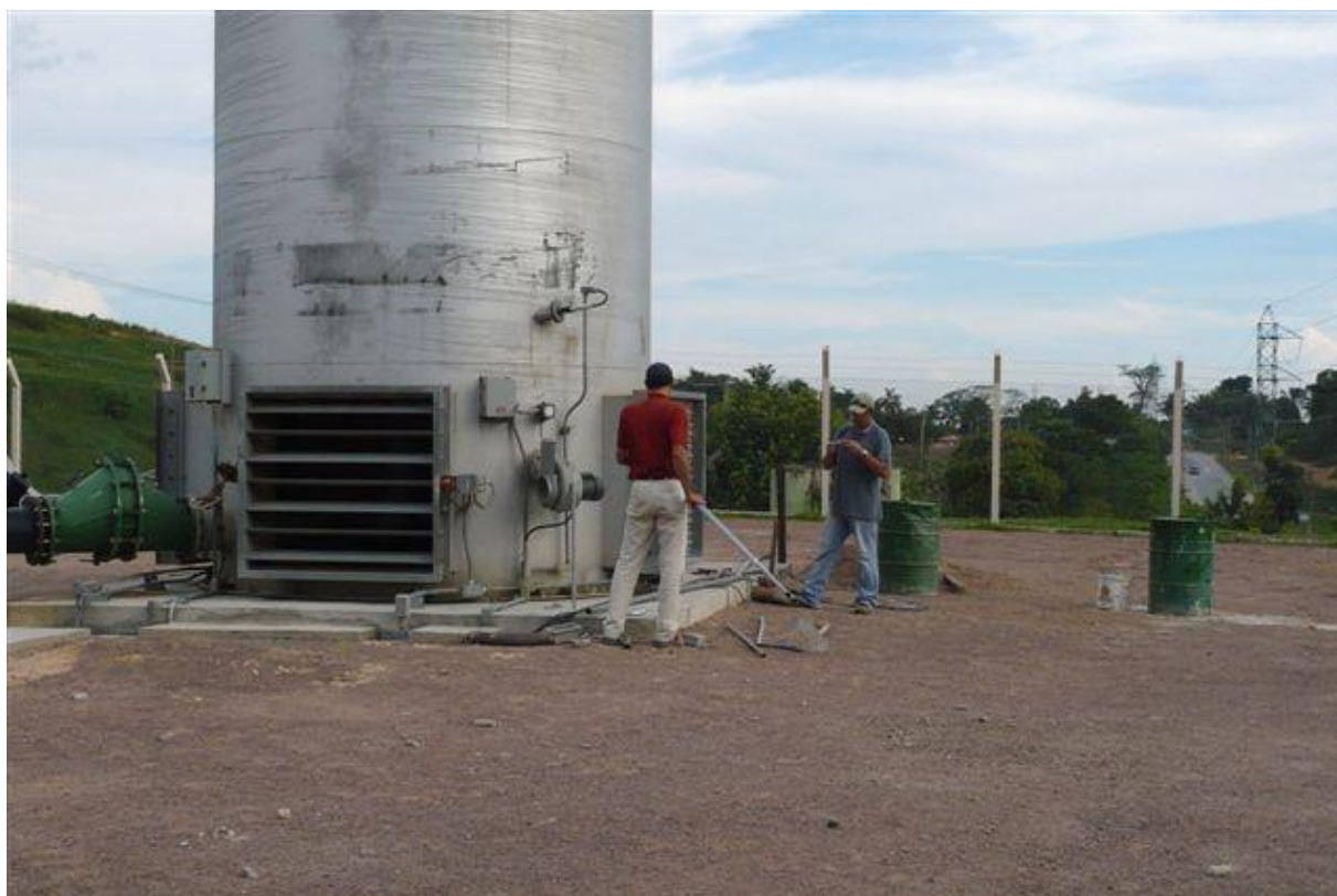
Figure 8 - Detail of Enclosed Flare
