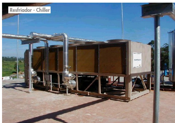
Figure 9. Example of Absorption Chiller (source: Biogás Ambiental, accessed on January 31 st , 2006 5 )
