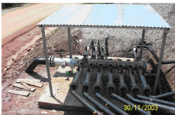
Figure 5. Example of manifold, connected to the transmission pipeline
