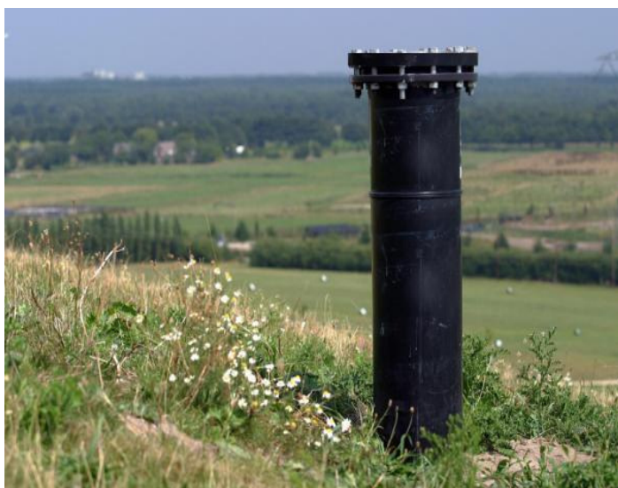
Figure 3. Example of wellhead
