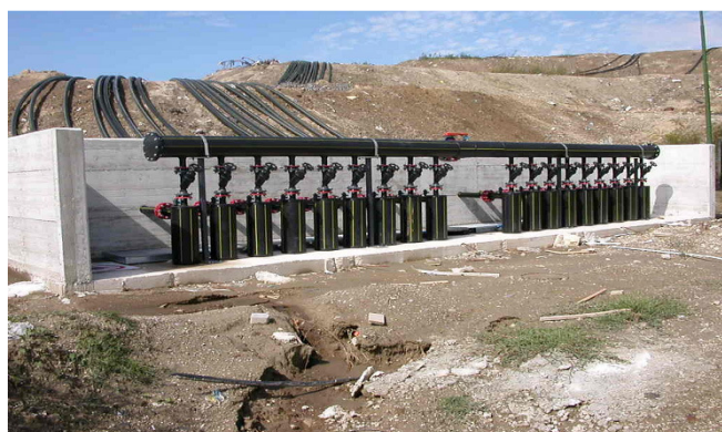
Figure 6. Example of Gas Regulation Station (source: Multiambiente, accessed on January 31 st , 2006 3 )
