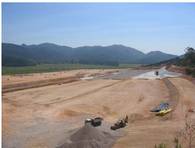
Figure 5: Installation of geomembrane on top of zone 1
