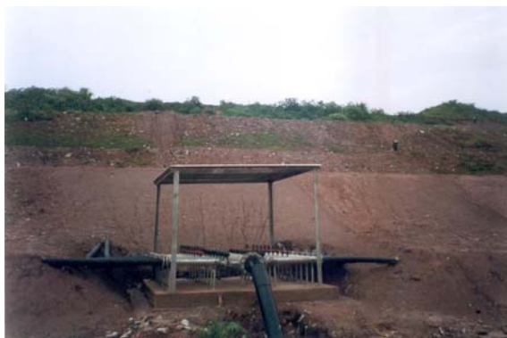
Figure 6. Example of manifold, connected with the transmission pipeline
