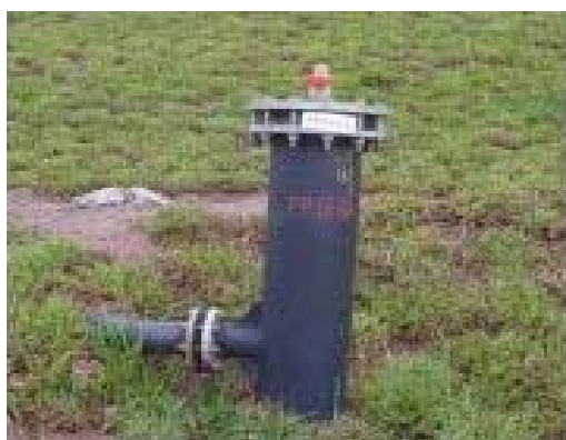
Figure 4. Example of wellhead (source: Biogás Ambiental 3 )
