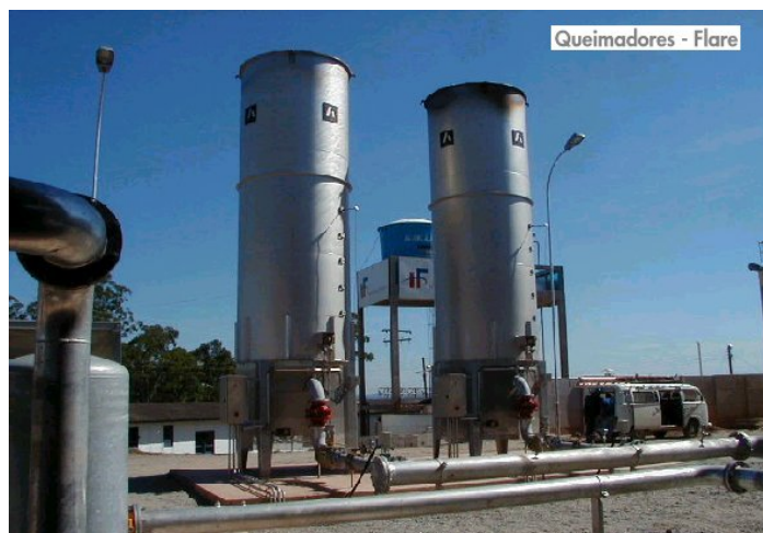
Figure 8. Example of flares (source: Biogás Ambiental)
