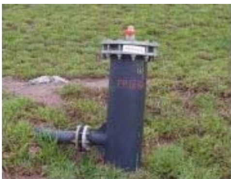
Figure 4. Example of wellhead (source: Biogás Ambiental 3 )
