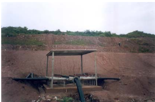
Figure 7. Example of manifold, connected to the transmission pipeline
