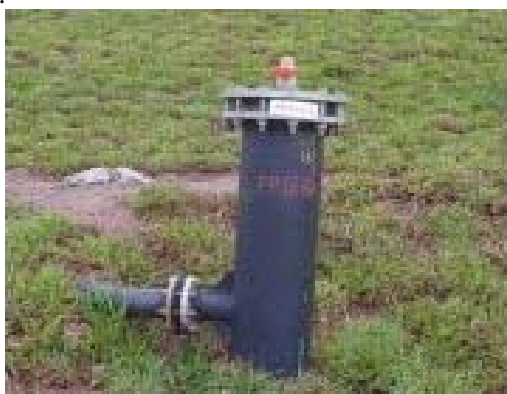
Figure 3. Example of wellhead (source: Biogás Ambiental 4 )
