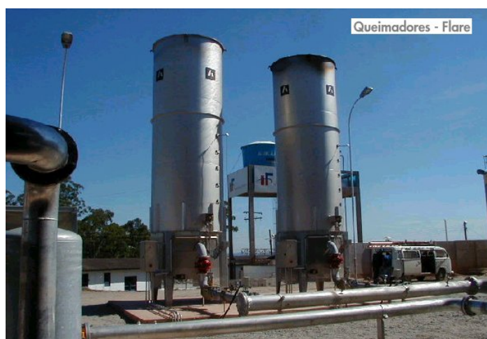
Figure 7. Example of flares (source: Biogás Ambiental)
