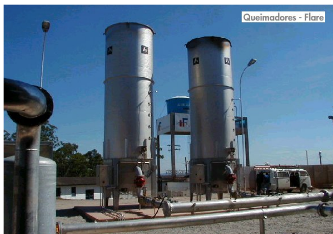
Figure 7. Example of flares (source: Biogás Ambiental)
