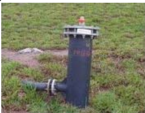
Figure 3. Example of wellhead (source: Biogás Ambiental 4 )
