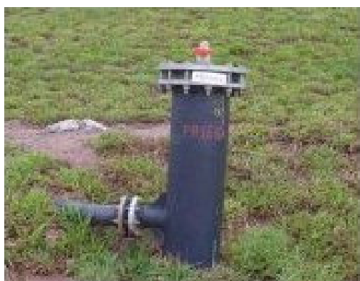
Figure 3. Example of wellhead (source: Biogás Ambiental 5 )
