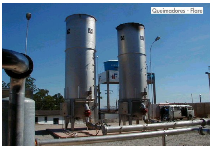
Figure 7. Example of flares (source: Biogás Ambiental)
