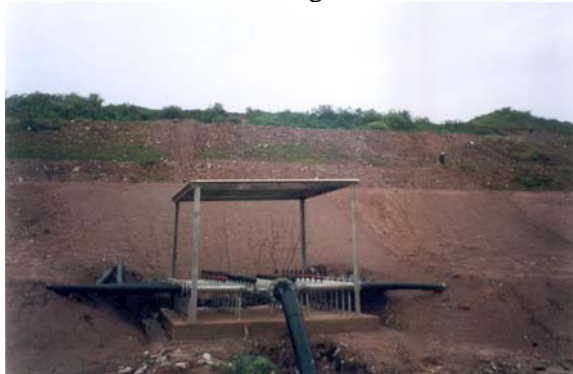
Figure 5. Example of manifold, connected with the transmission pipeline
