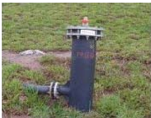
Figure 3. Example of wellhead (source: Biogás Ambiental 4 )
