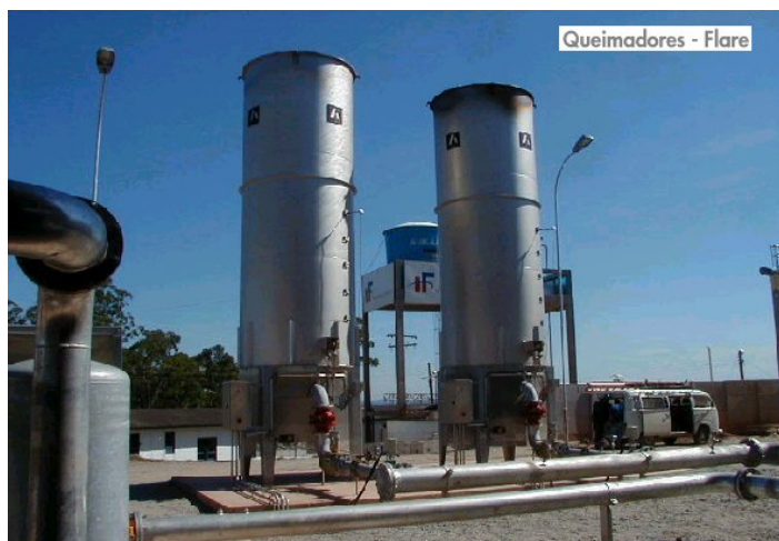
Figure 7. Example of flares (source: Biogás Ambiental)
