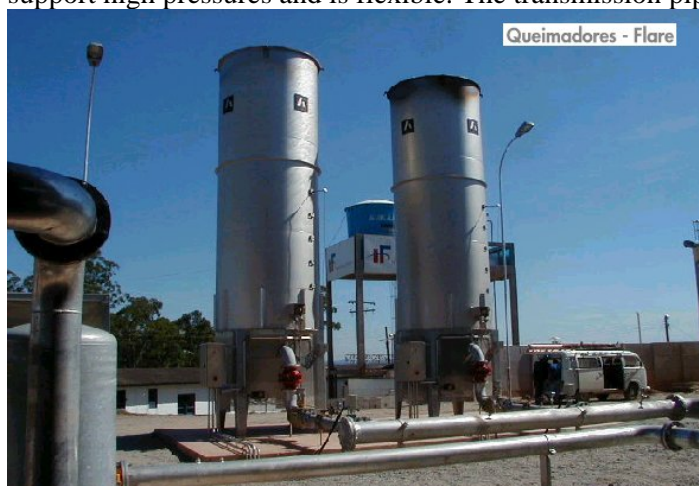
Figure 7. Example of flares (source: Biogás Ambiental)
