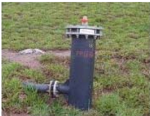
Figure 3. Example of wellhead (source: Biogás Ambiental 4 )
