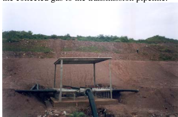
Figure 5. Example of manifold, connected with the transmission pipeline
