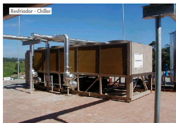
Figure 11. Example of Absorption Chiller (source: Biogás Ambiental, accessed on January 31 st , 2006 8 )
