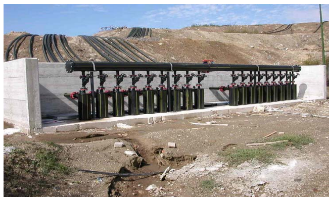
Figure 8. Example of Gas Regulation Station (source: Multiambiente, accessed on January 31 st , 2006 6 )
