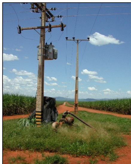
Figure 6: Example of one installed electric irrigation engine and new transmission line designed exclusively for irrigation activities.
