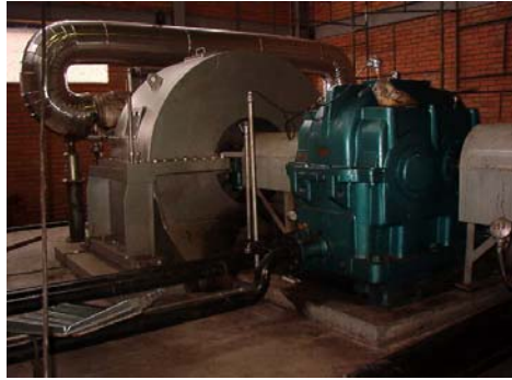
Figure 5: Dresser Hand turbine, with 10 MW of installed capacity.
